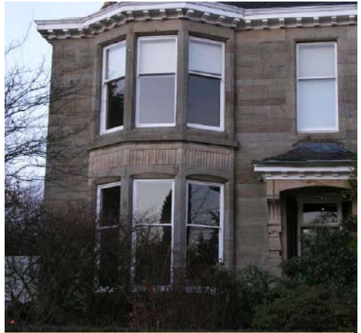
Stanley: The decorative masonry to window bay panels and porch support columns contributes to the character.
